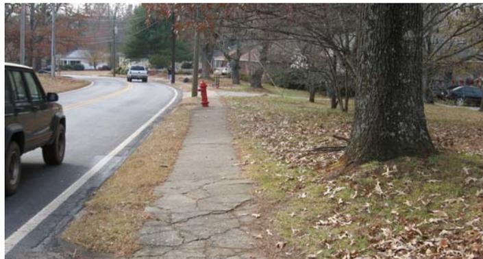
*Sidewalks on Wayside Street are in poor condition and objects within the path of travel make them non compliant with ADA standards*
