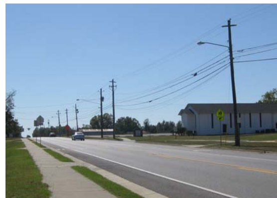
The midblock crossing in front of the school is difficult to see.
