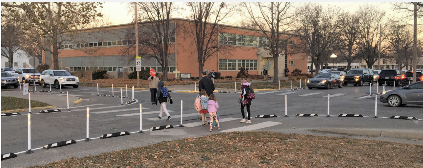
Students wait in right-of-way protected by rubber curbs and bollards before crossing the street to school in Manhattan, KS—photo from Flint Hills MPO.
