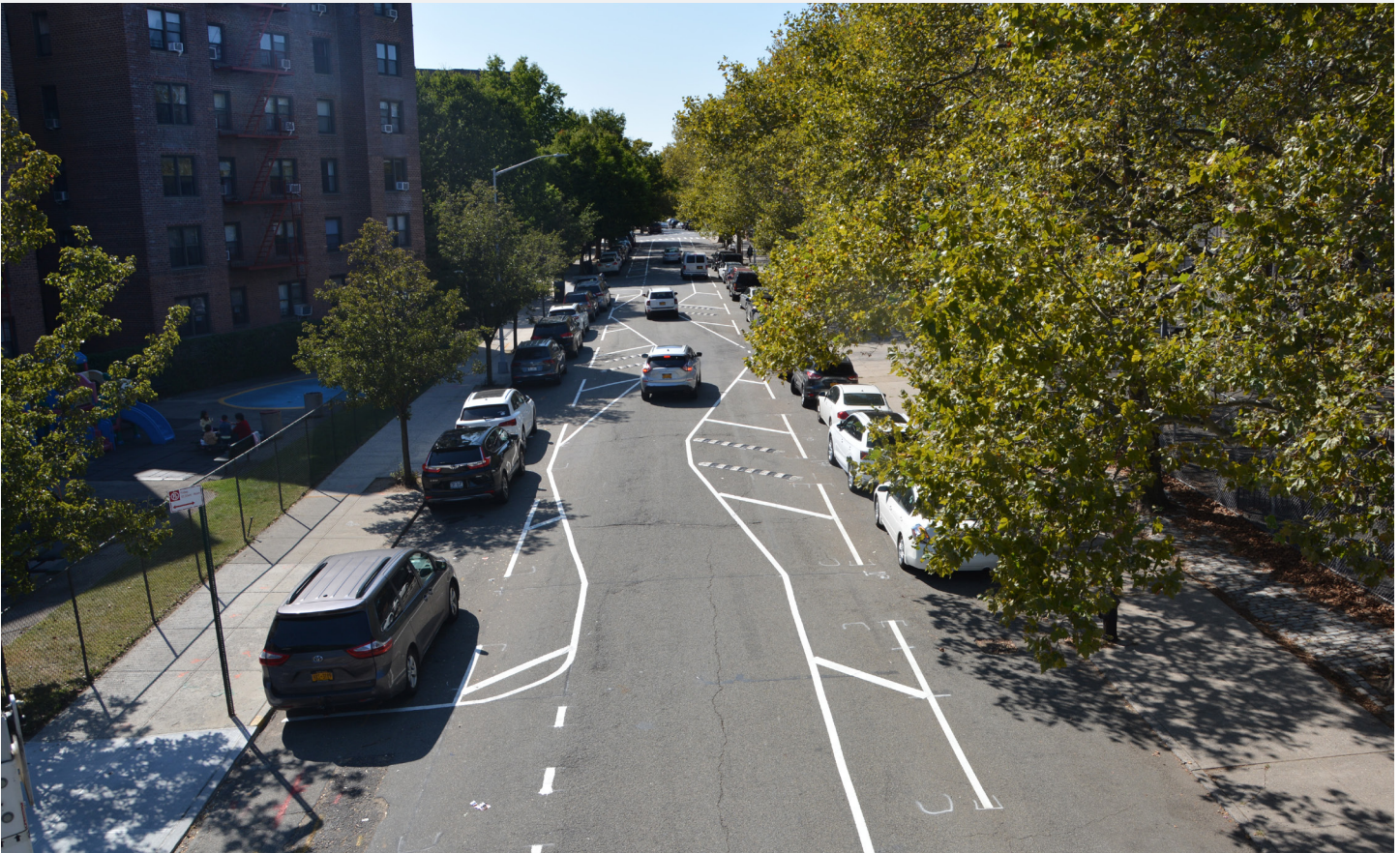
Chicane along 71st Avenue in Queens. Photo provided by NYC DOT.
