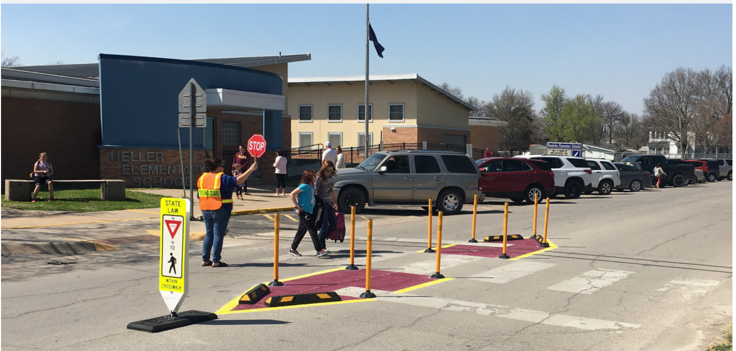
Pedestrian refuge island installed at Heller Elementary School in Neodesha, Kansas.
