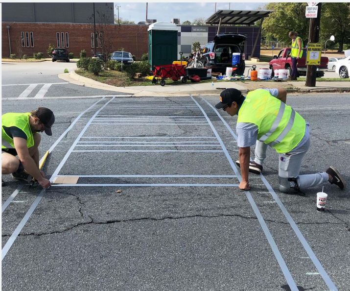
Volunteers install a high visibility crosswalk in Macon, GA using reflective tape. Photo provided by Bike Walk Macon.
