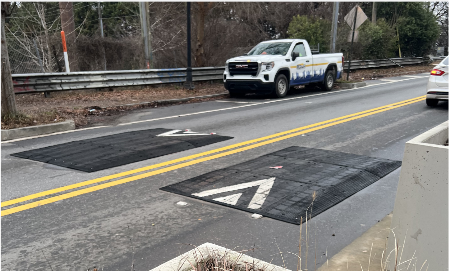
Speed cushions installed on the Atlanta Beltline just south of Moreland Ave in Atlanta, Georgia. Photo by: Ron Knezevich.
